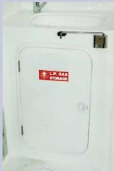
Warning labels should be displayed next to the cylinder and appliance
