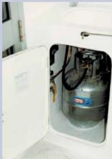
Warning labels should be displayed next to the cylinder and appliance
